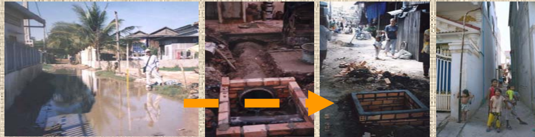
Roads and drainage improvement
